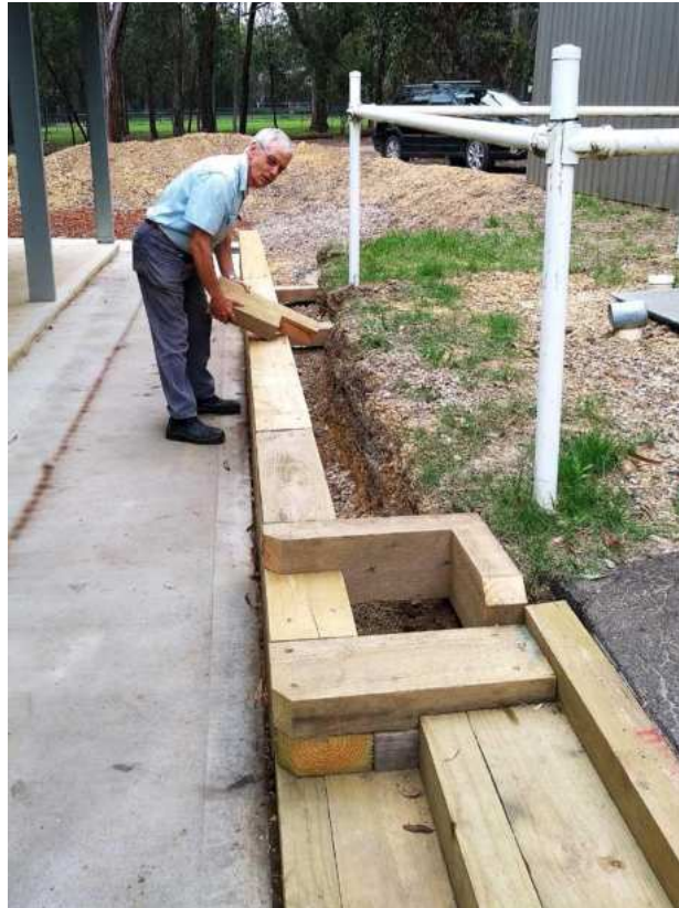
Malcolm is working on the retaining wall between our extension and the Douglas Pickering Pavilion. When the wall is in place the remaining rubble pile at the back of the extension will be used to backfill the space.
